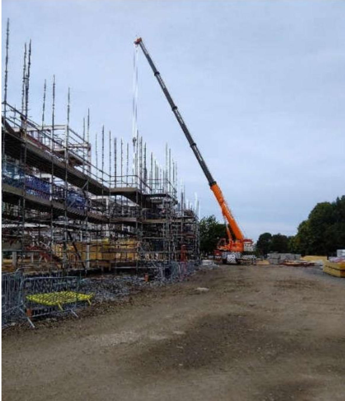
Travelling crane lifting in timber kit panels and plasterboard
