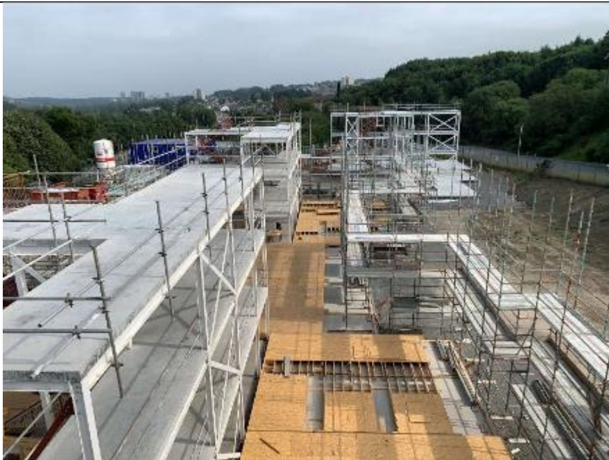
Scaffold erection to Block B
